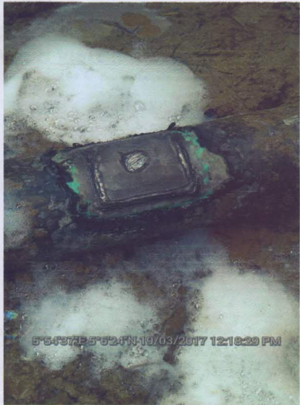
INCIDENT POINT AFTER REPAIR
